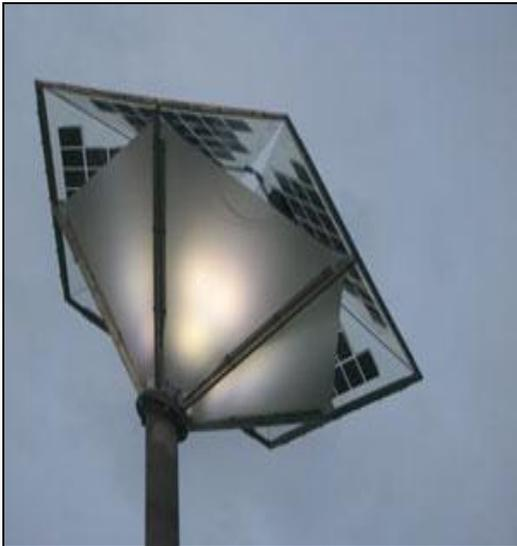
PICTURE 16: New photovoltaic street lamps.
